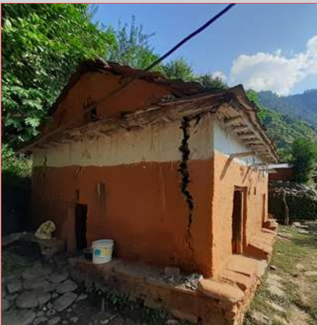
Figure 4. Houses with large cracks in Kuch Village
