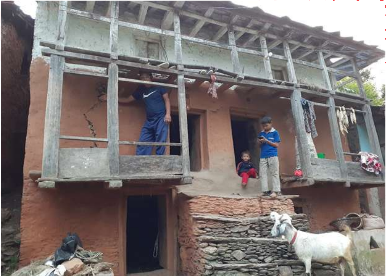
Figure 7. Traditional houses to accommodate livestock on the ground floor
